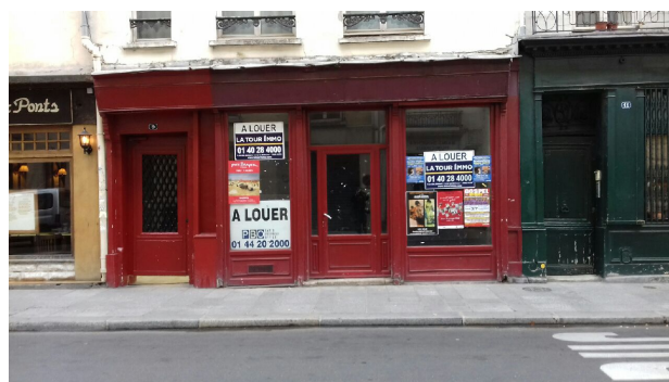
Local commercial vacant – Paris 4 e © DRIEA – Salagnac – 2018
