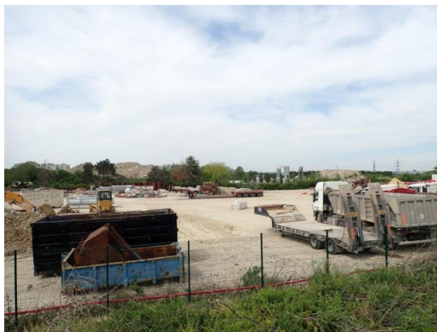
FIGURE 61: SITE INDUSTRIEL @EGIS 2020
