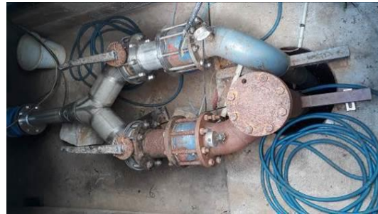
Figure 4 : Photo tête forage
