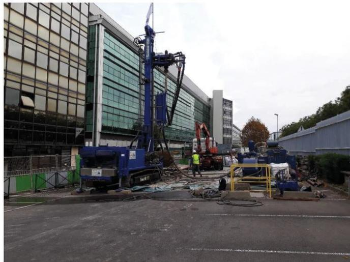
FIGURE 12 : PHOTO D'UNE MACHINE DE FORAGE ET DE SES EQUIPEMENTS PERIPHERIQUES
